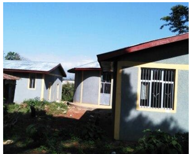
Youth center construction, Waktola Guedeta
